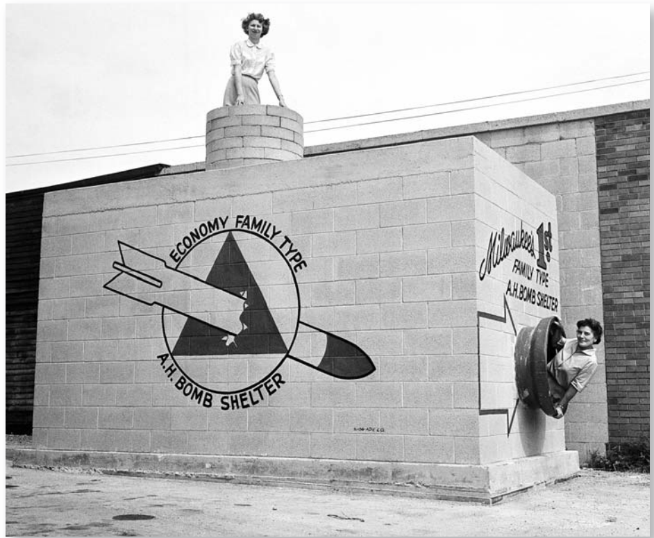
(L-R) Beverly Wysocki and Marie Graskamp emerged from a new family-type bomb shelter on display in Milwaukee Sept. 12, 1958. The shelter measured 8 feet by 8 feet by 14 feet 8 inches high and could hold eight to 12 persons in an emergency. It could be buried in the earth for added protection. Covered with 3 feet of earth, it was said that the shelter would be safe to within three quarters of a mile of ground zero if a 20 megaton nuclear bomb were to be dropped. The price ranged from $1,300 to $1,400 installed.
